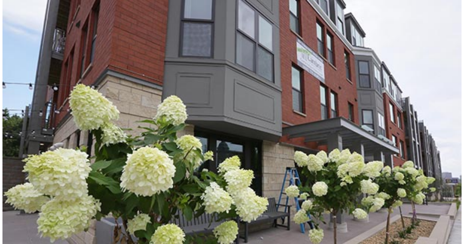
Dominium is putting the finishing touches on The Cambric, a 113-unit senior project at 720 E. Seventh St. in St. Paul. (Staff photo: Bill Klotz)
